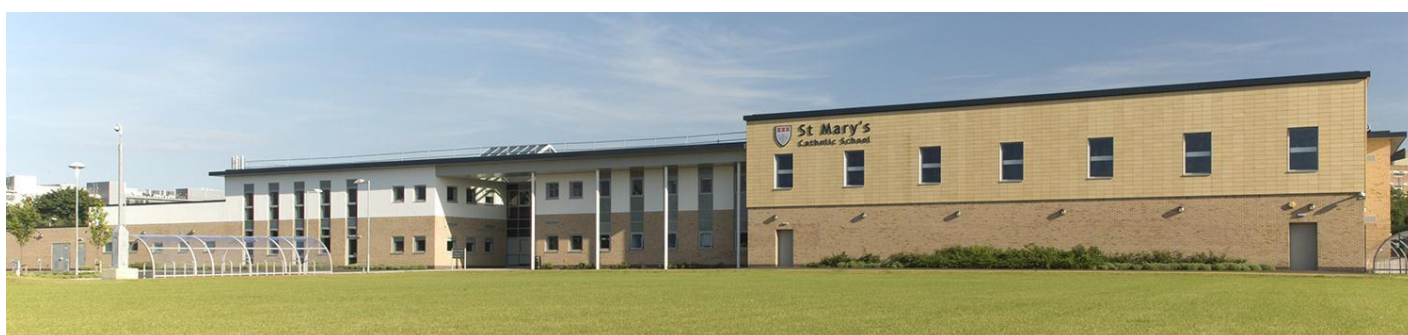
The school – front view
